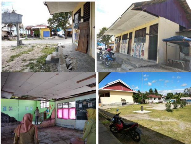
The pictures of the school after the earthquake
